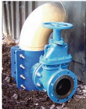
Install the valve to the clamp ready for pressure testing
