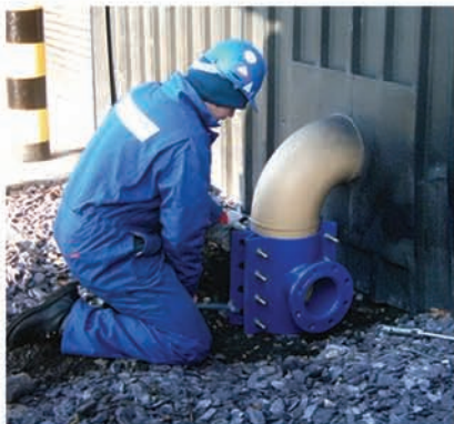
Firstly secure the clamp around the pipe where the valve is to be fitted
