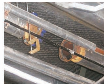
Only when the freeze(s) have been confirmed is work allowed to be carried out
